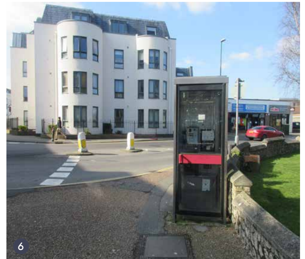
Phonebox in state of disrepair juxtaposed with exposed paving aggregates and the church wall.
