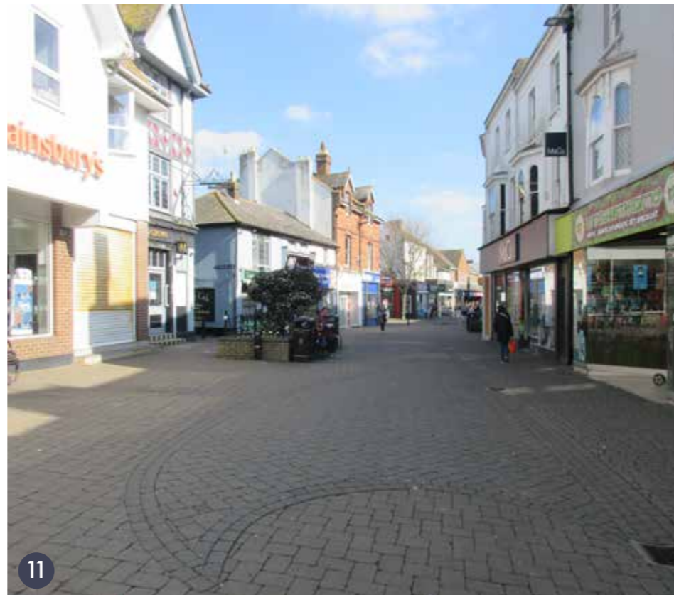
11 Existing block paving has proved resilient to 30 years of High Street traffic.
