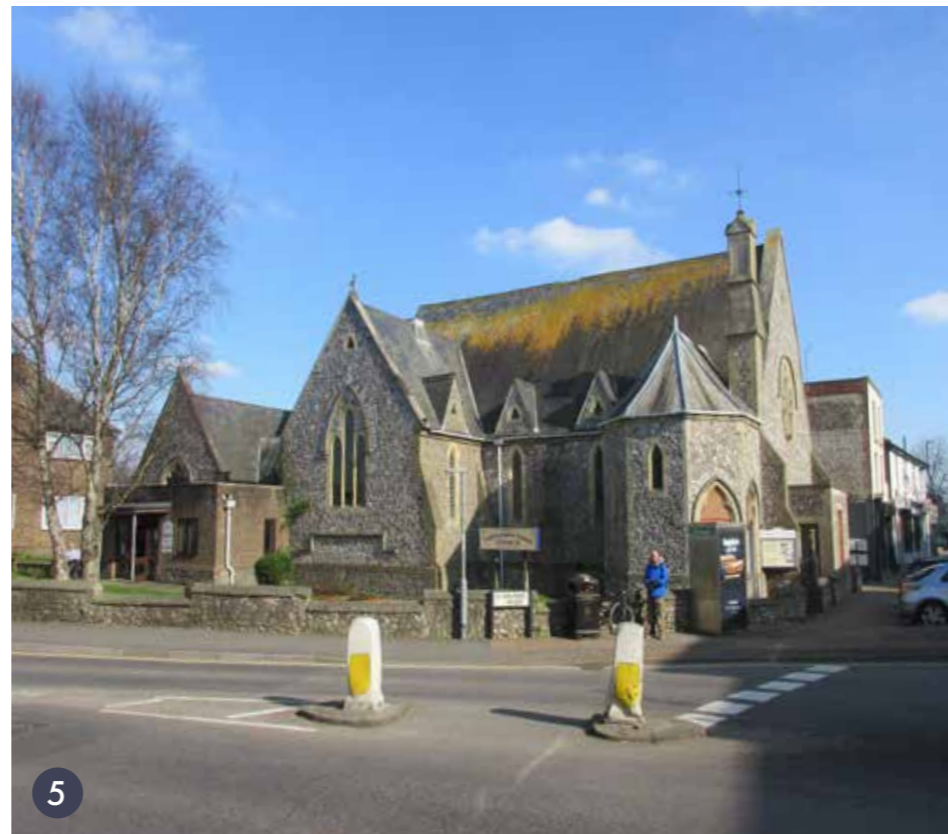
Littlehampton United Church: a recognisable landmark, not least for the use of vernacular materials.
